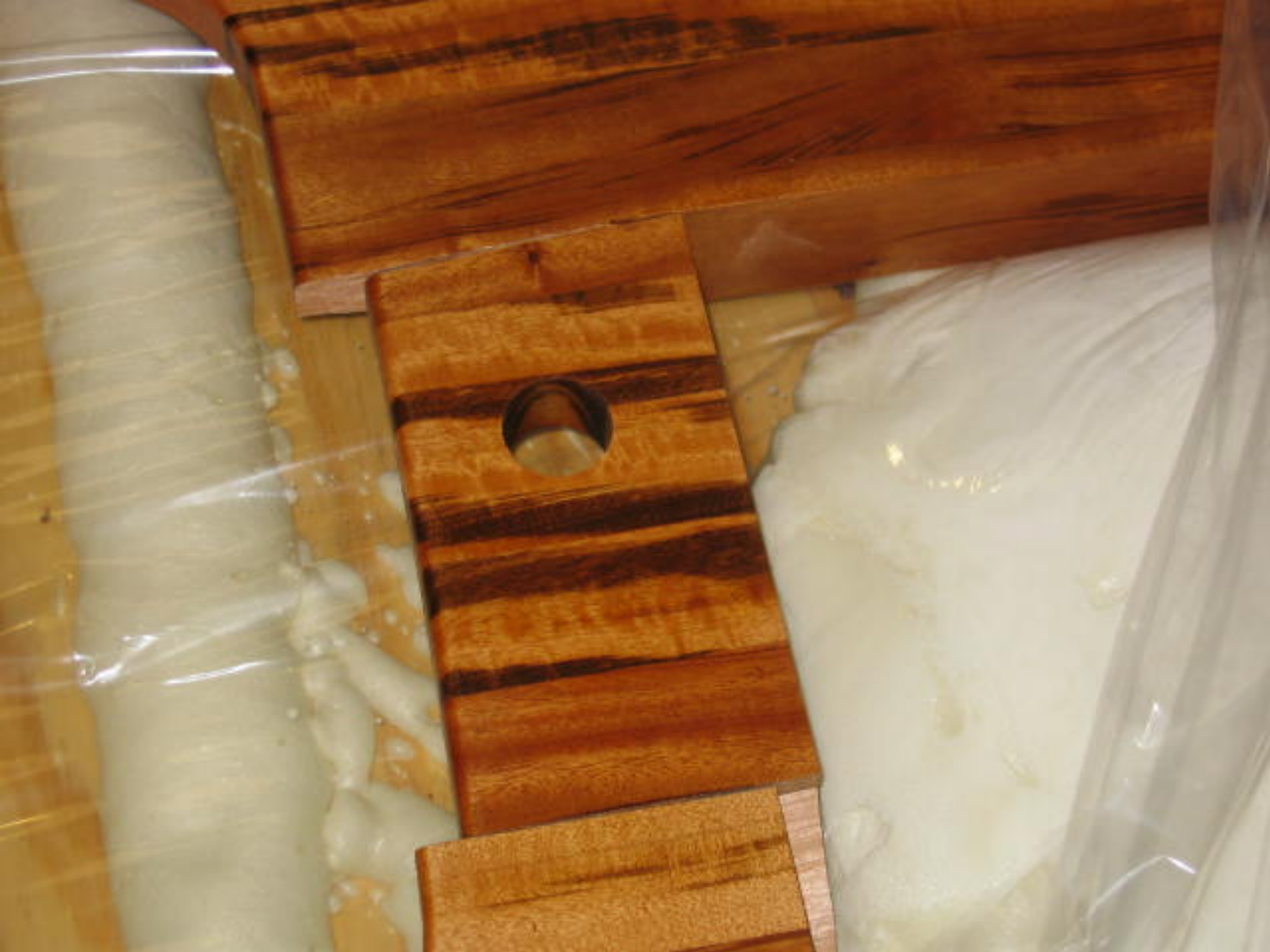
Picture Number: 6 of 8 For CPFC Pro #: DEMOINSPECTION022206 CPFC_DEMOINSPECTION022206_pic_6.jpg
